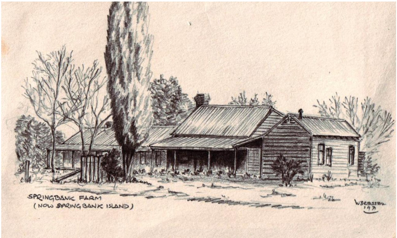
Springbank Farm – now Springbank Island (1971)
