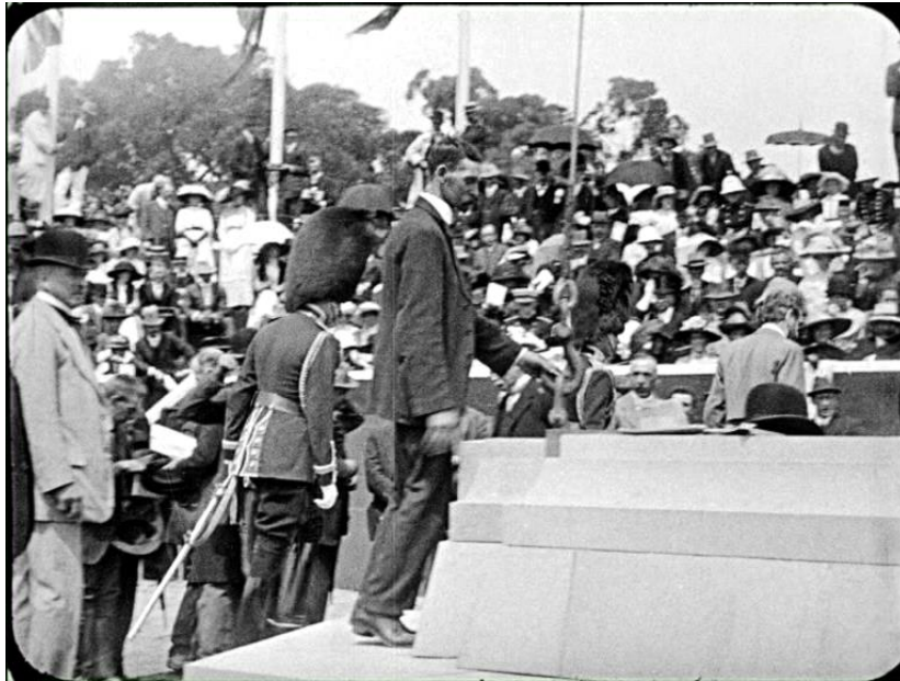
The man standing on the stones is Fred Young supervising the commencement column stones being placed on 12 March 1913. Source: Michael Hall.
